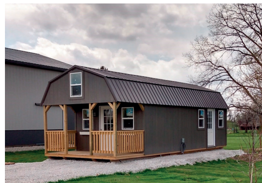
12'x32' Driftwood Urethane (LP) SmartSide (LP) SmartSide (LP); Burnished Slate Metal Roof. (Shown with insulated windows & white flower boxes.)
