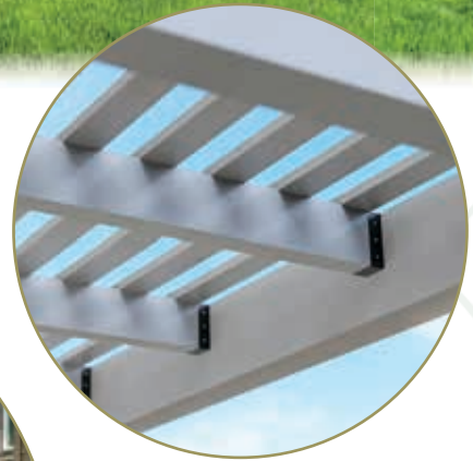
JOISTS AND PURLINS Underside of Roof
